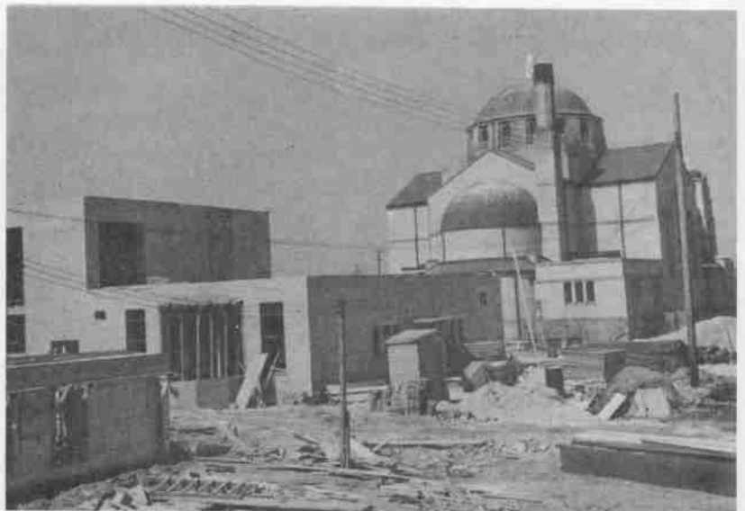
A scene of progress in the life of our parish...the erection of the parochial grade school.
