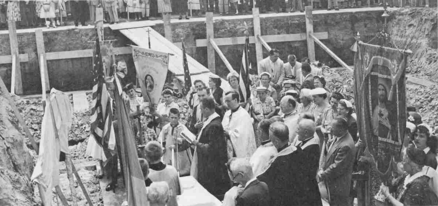
The ground is broken for the construction of a new rectory.
