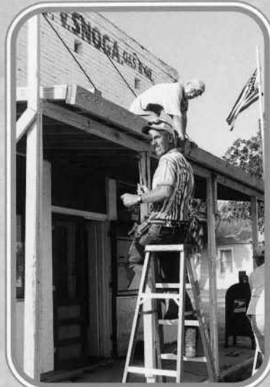
REPAIRING SNOGA'S STORE
