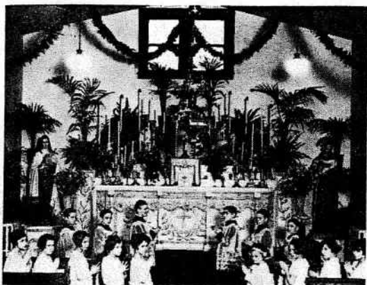
Sanctuary view before 1941
