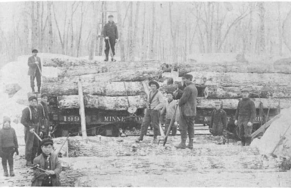
LEFT: Loggers of all ages pause from loading logs on railroad cars to have their picture taken.
