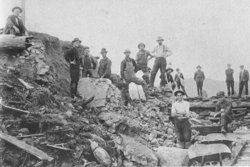
LEFT: Construction of an early bridge over M-75. Some of the workers were: Mr. Meeker, Mr. Dixon, Mr. Nelson, John Baker, Mr. Knudson, Leo Grobaski, Jake Fike, George Smith, Rupert Porter, Mr. Moyer, Albert Worthing and Harry Walker.
