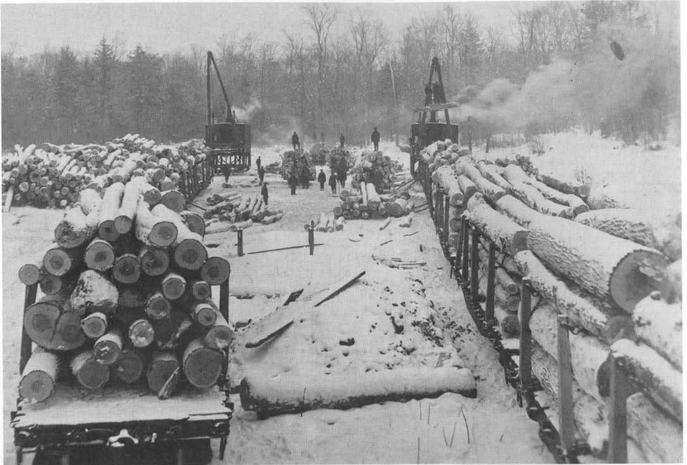
This winter scene of the Cobb and Mitchell Camp demonstrates the loading of logs for transporting to mills by railroad.
