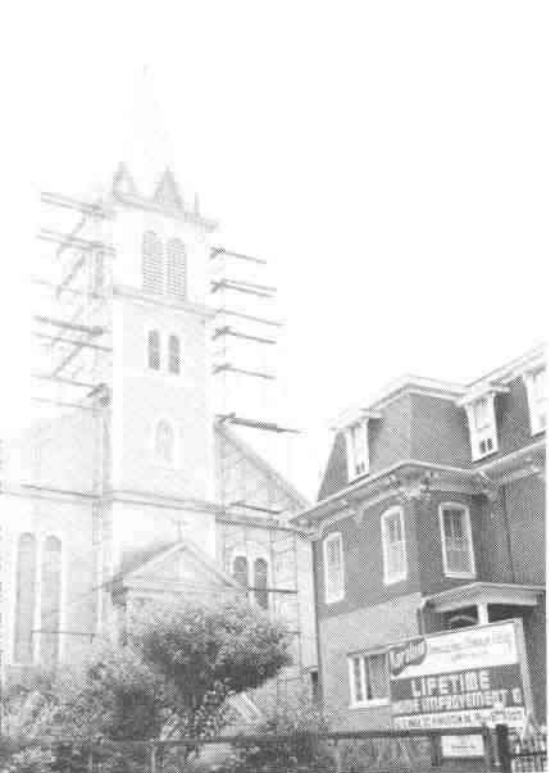
Scaffolds for aluminum siding
