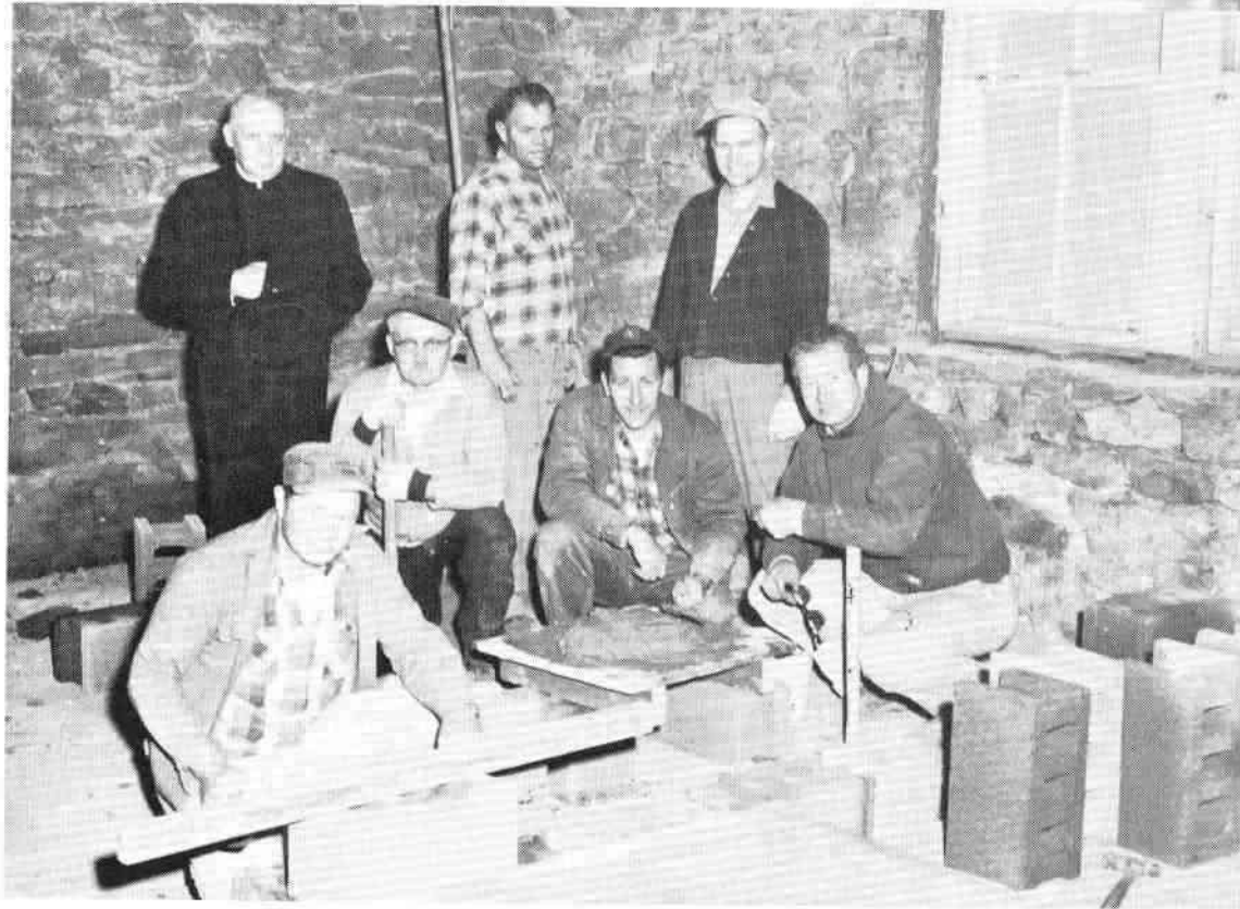
Beginning of Renovation in Auditorium 1967
