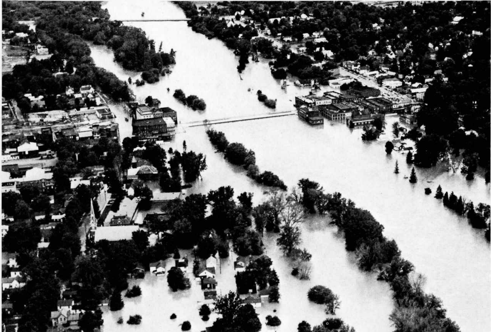
FLOODED SALAMANCA — Water from Allegheny River pours over downtown Salamanca during Friday's record flood. This aerial photo, taken in midmorning, shows Main St. bridge in foreground and Parkway Bridge farther up river. Dikes and floodwalls along both banks of the river are covered by water, which rose 72 feet above previous flood record here. This is one of a series of aerial photos of the flood made by a member of the Salamanca Republican-Press staff. Other aerial photos are on pages 6 and 7.
