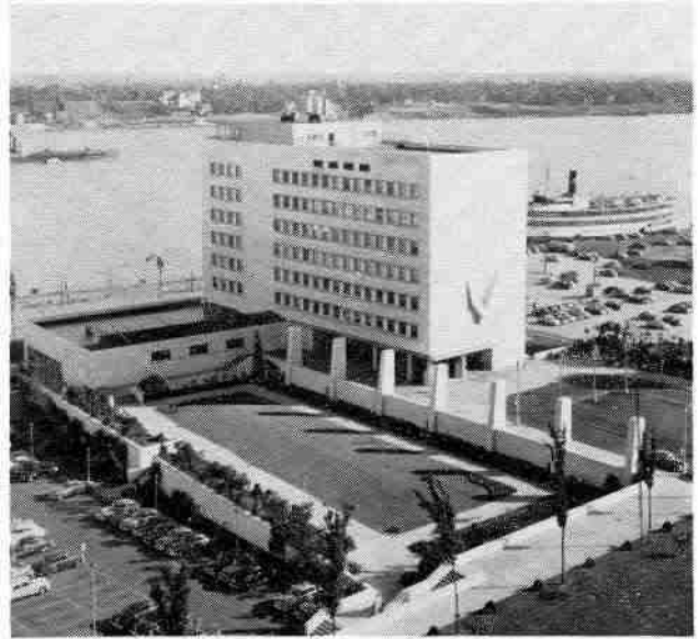
The VETERAN'S MEMORIAL, completed in 1950, is the first building in the beautiful new Civic Center which is taking shape along Detroit's Riverfront. Its ten floors of auditoriums and meeting rooms are in constant use by civic and veterans' organizations. The massive eagle ornament was designed by sculptor Marshall Fredericks.
