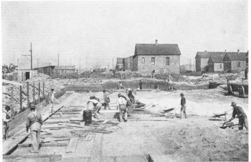
Parishioners began laying the foundation of the present site of SS. Peter and Paul Church in 1906.
