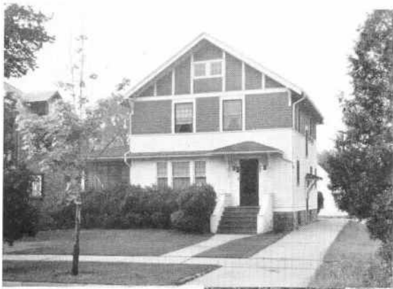
PLATE 4 View of the Original Rectory on Houstonia Avenue
