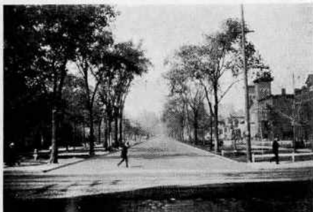
OLD WASHINGTON AVENUE, WITH THE FORMER ST. ALOYSIUS CHURCH ON THE RIGHT
