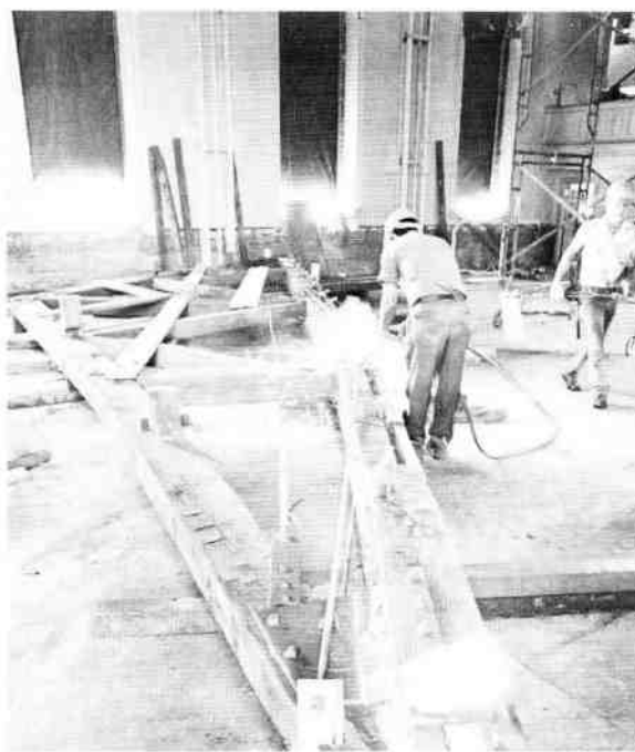
Original black walnut structural beams. July 30, 1987. (Courtesy Monroe Evening News.)
