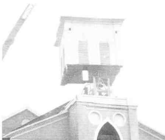
Removal of old tower (Photo taken by Lynn Reaume.)
