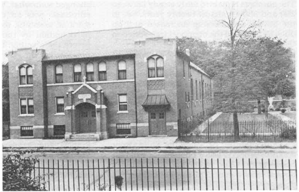
New Third Order Hall completed
