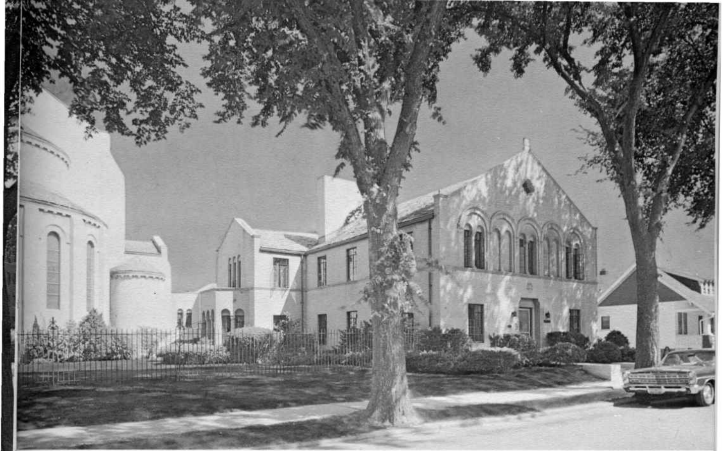
The beautiful white edifice that serves as a Rectory is amply supplied with windows that allow its inhabitants the inspiration of communion with God's miracles of nature
