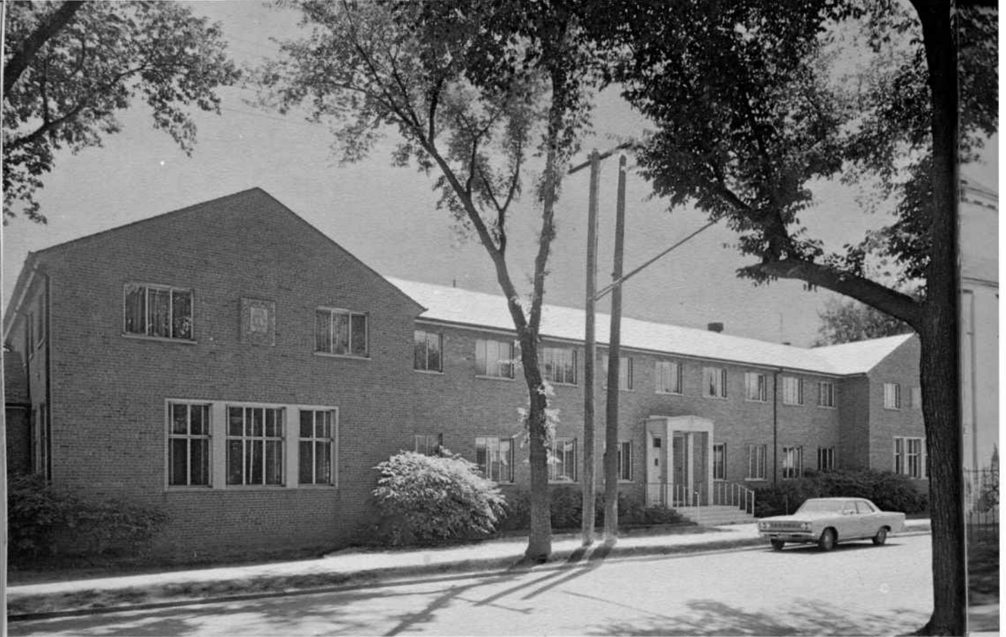
St. Cecilia's Convent is a trim brick building designed for ease of maintenance
