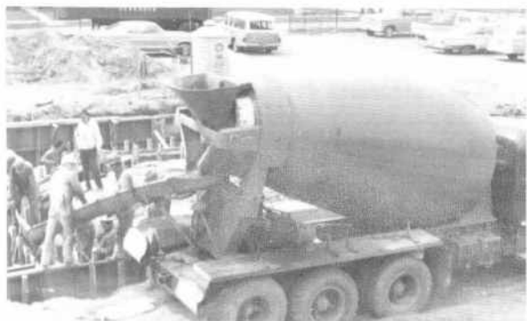
Construction of New Church.
