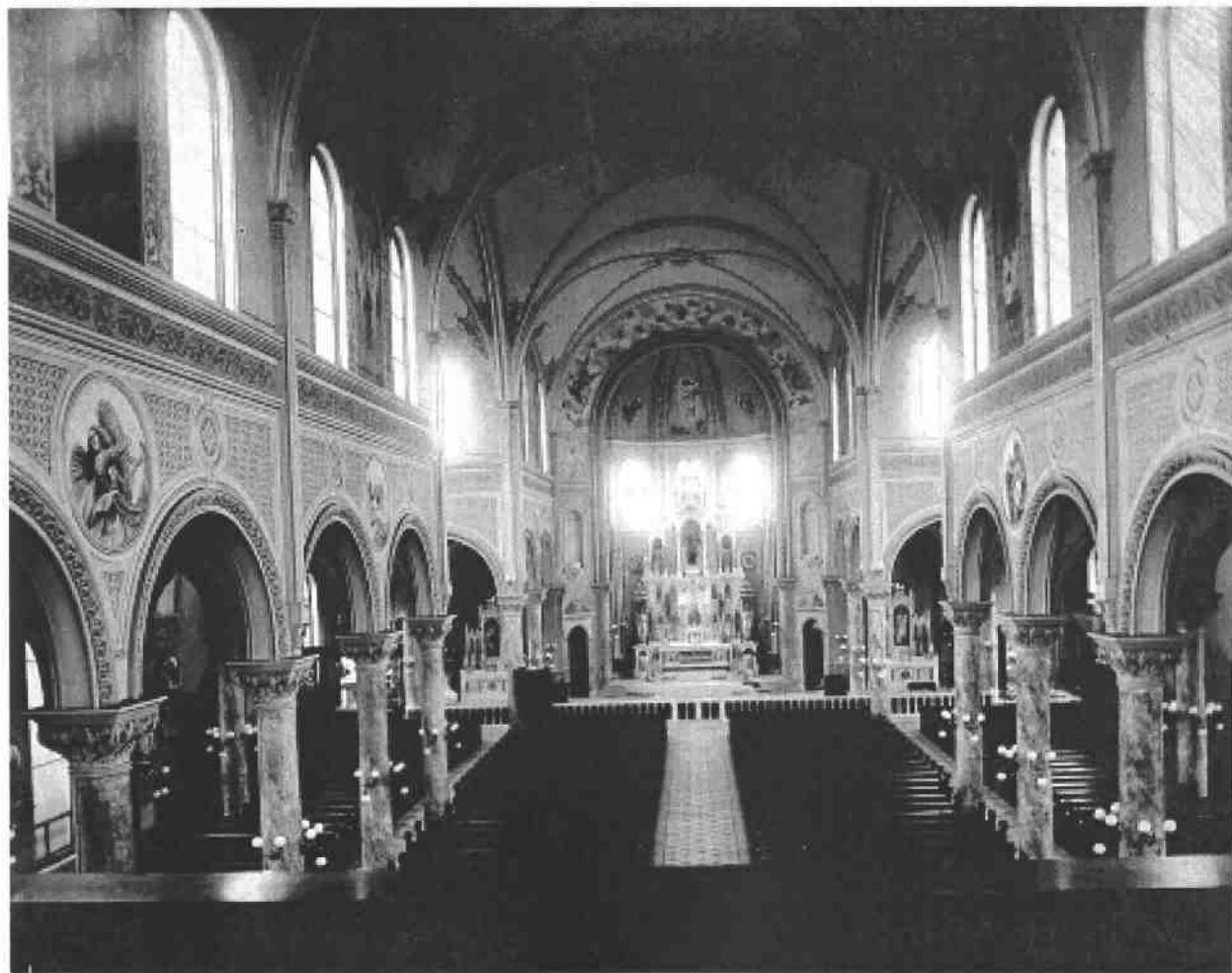
BELOW: INTERIOR OF THE NEW CHURCH - CIRCA 1917
