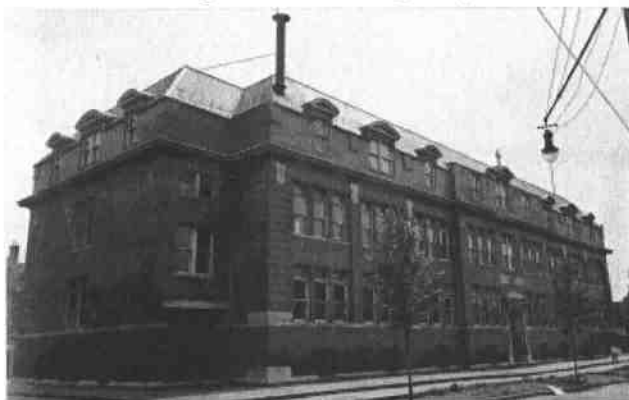
ST. HEDWIG STREET SCHOOL BLDG const. 1919, Architect: Harry J. Rill
