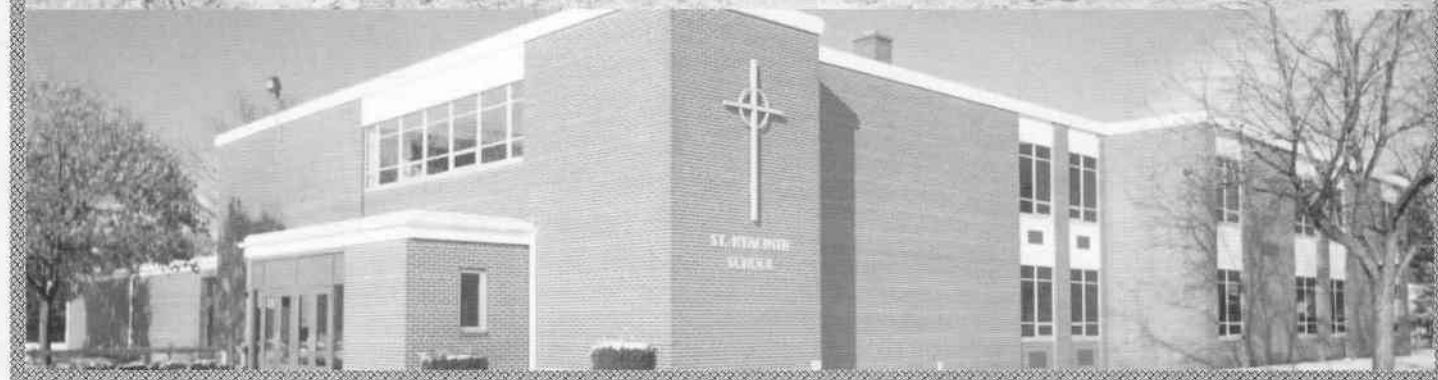
Breaking Ground for St. Hyacinth New Gym Building on July 17, 1966
