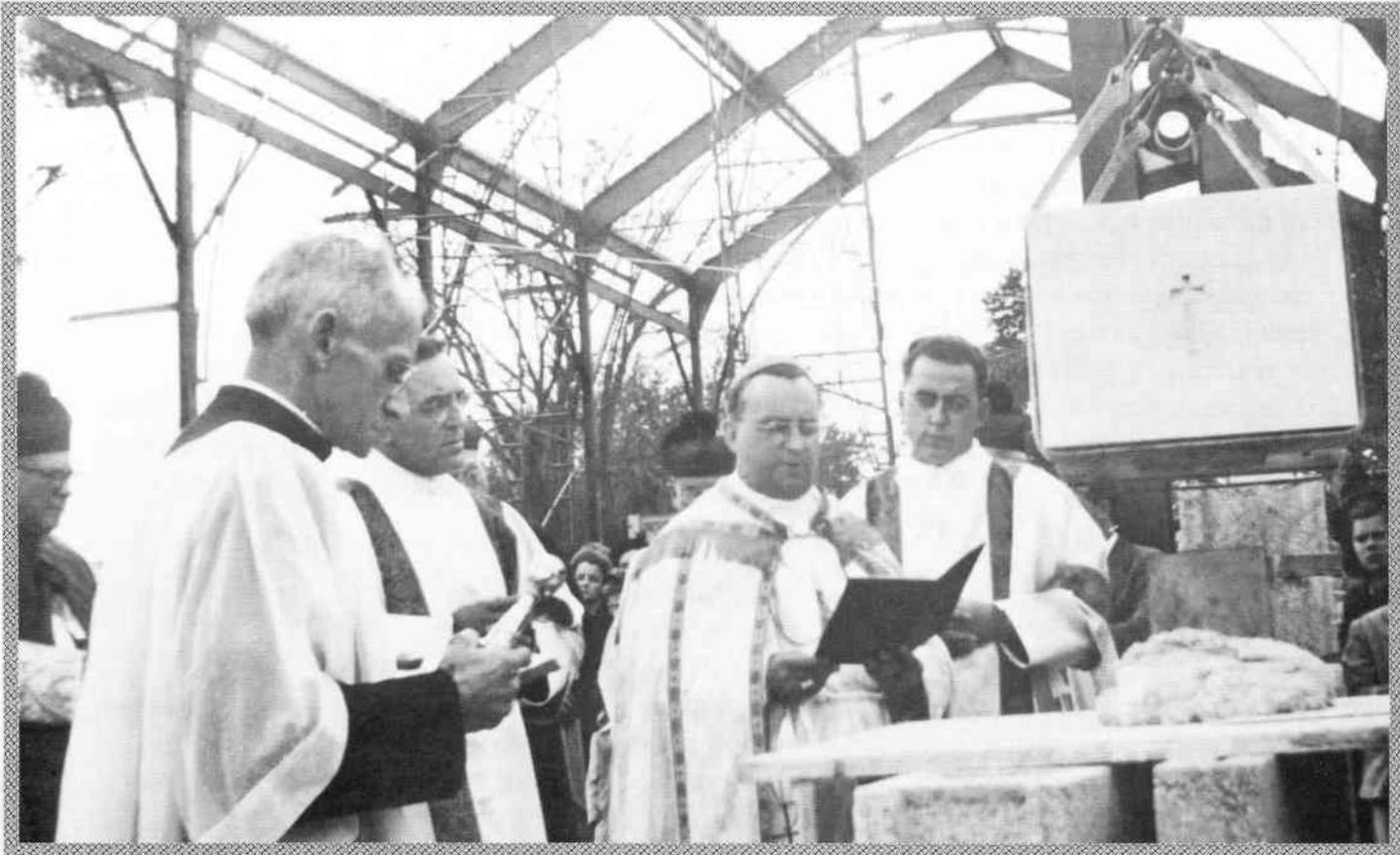
Laying of the Cornerstone for the new St. Hyacinth Church – October 8, 1950
