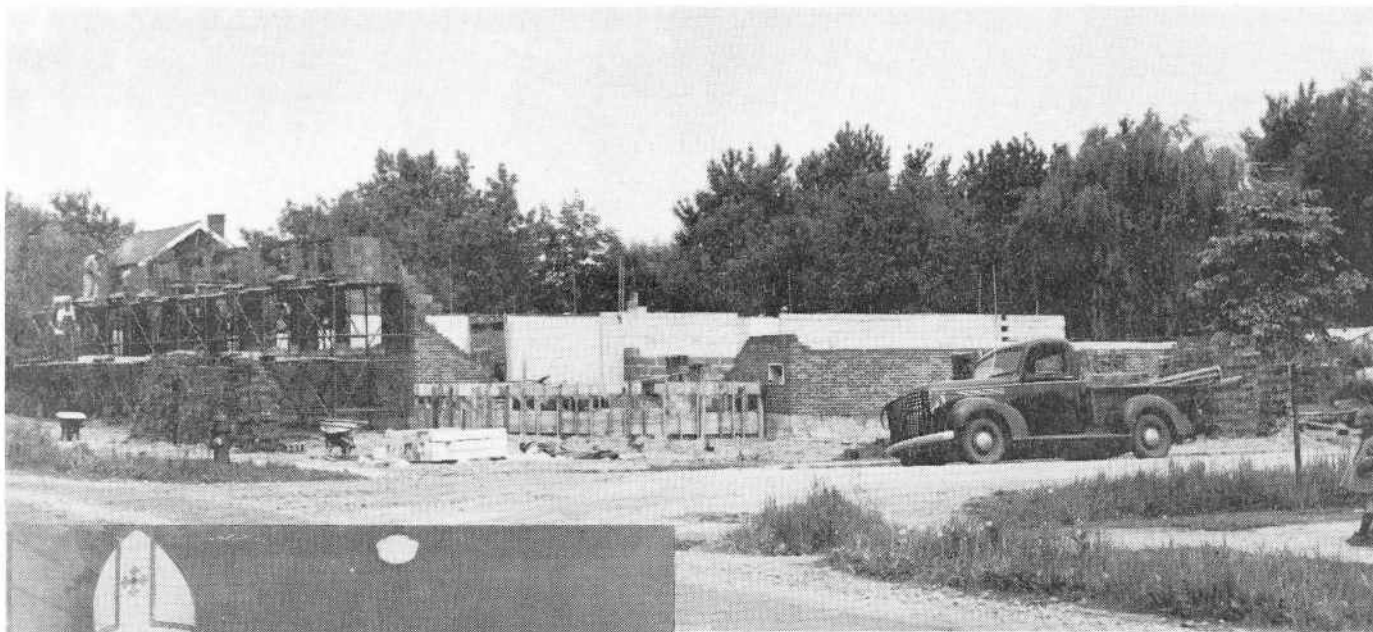
View of progress on building of new school - 1948.
