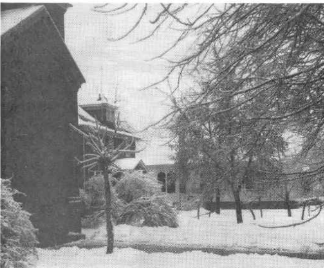
Entrance of School, center Rectory, Church
