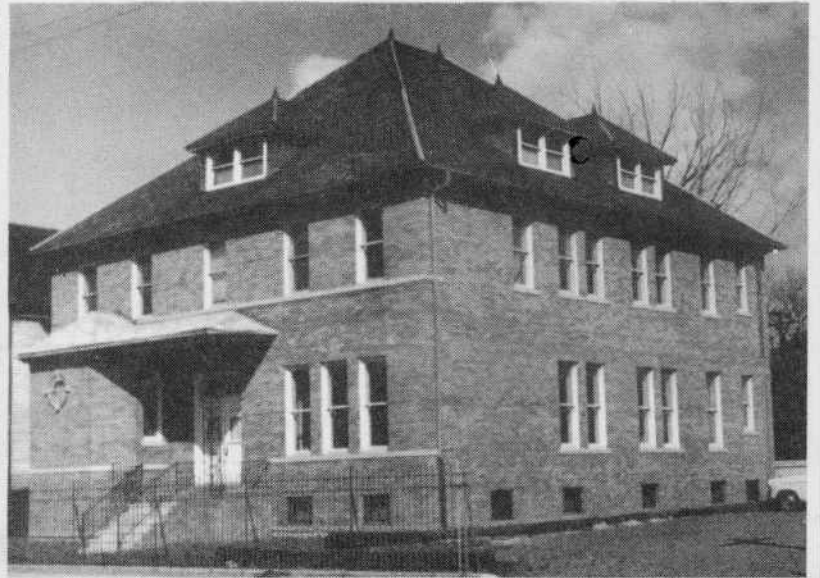
Before and After Sandblasting and Restoration
