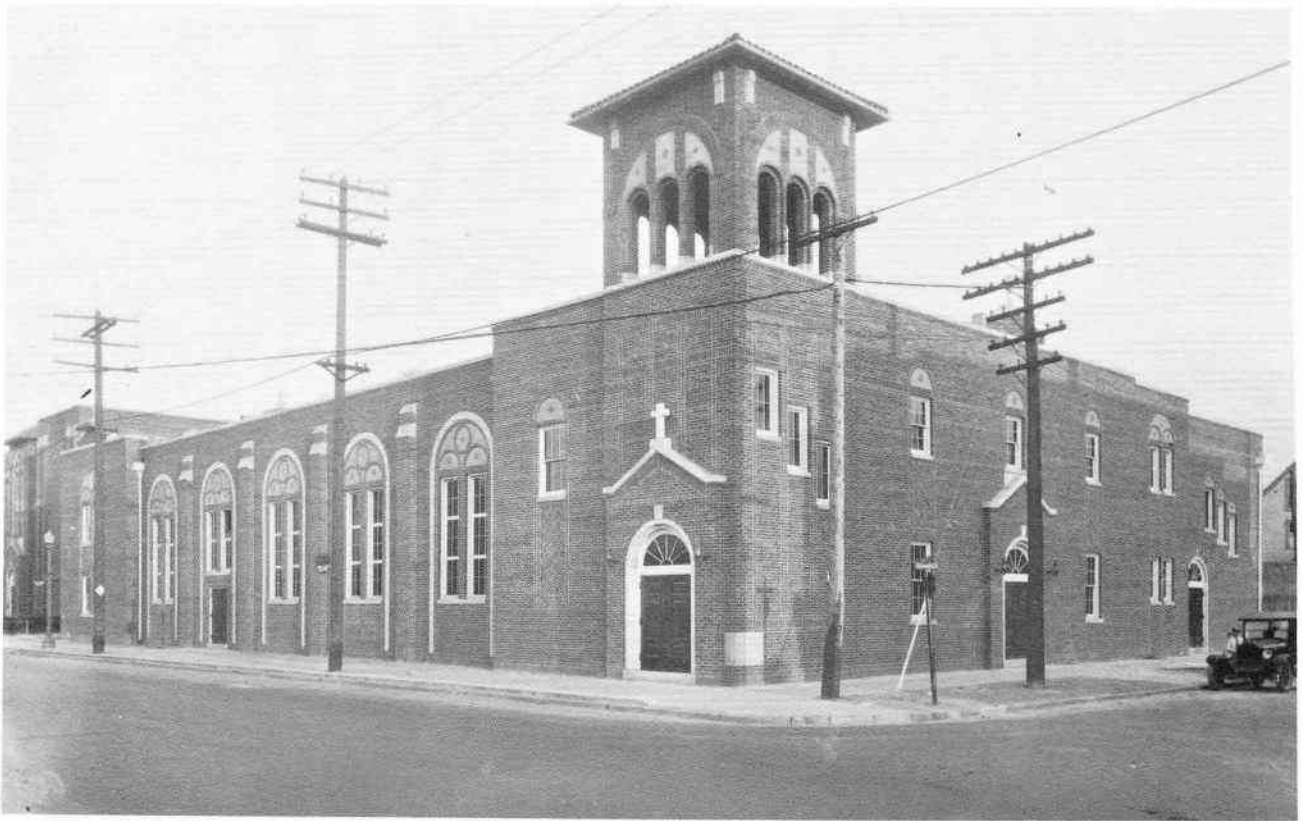
THE SECOND CHURCH STRUCTURE BUILT IN THE PARISH. IT STOOD ON THE CORNER OF BROMBACH AND CANIFF AVENUES, AND WAS BUILT IN 1929-30.
