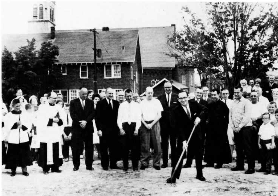
St. Mary's ground-breaking for new school, Sunday, July 31, 1966
