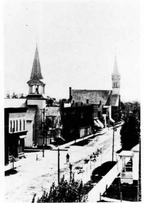
Dock St.-between Lake and Miller-rebuilt after fire of 1888 (Immanuel Lutheran Church and St. Mary's)
