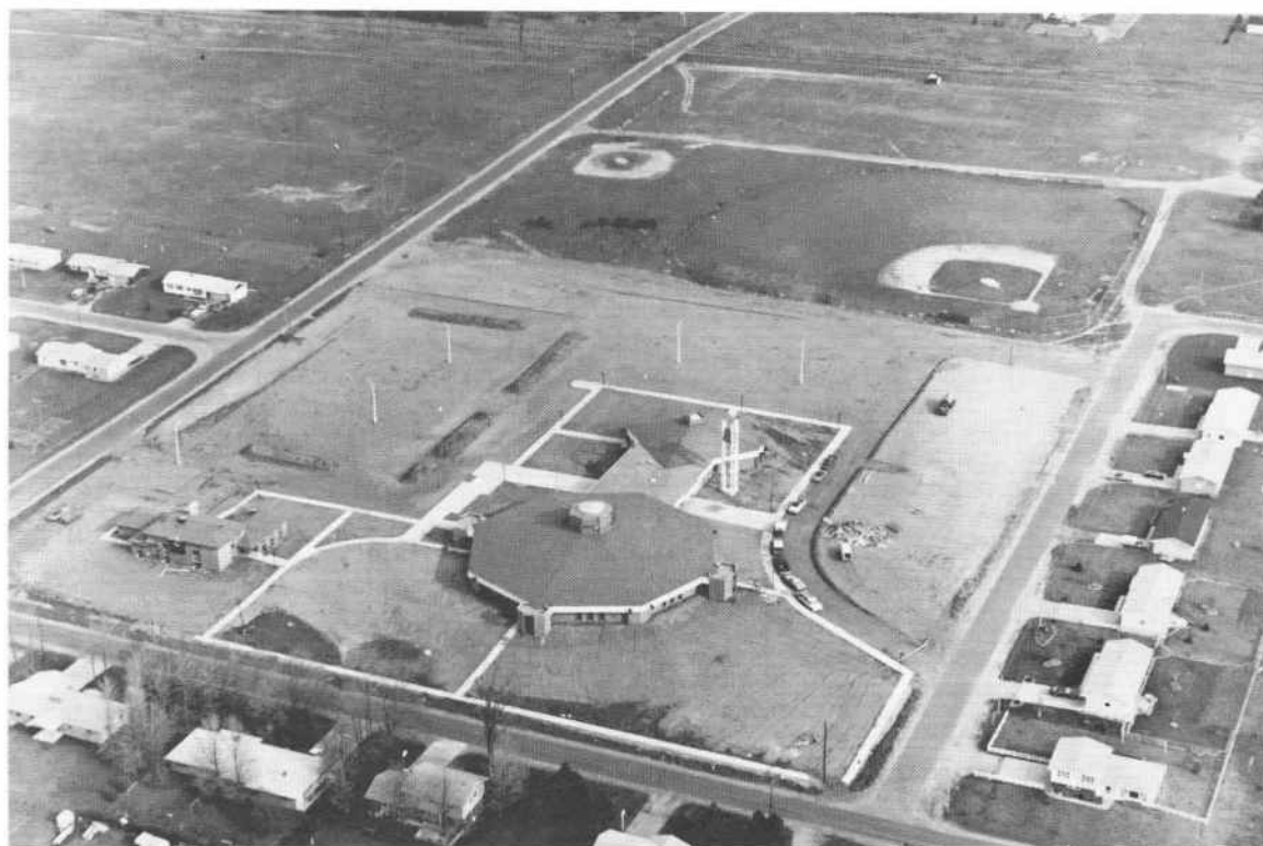
Aerial view of cathedral, hall and rectory as construction neared completion
