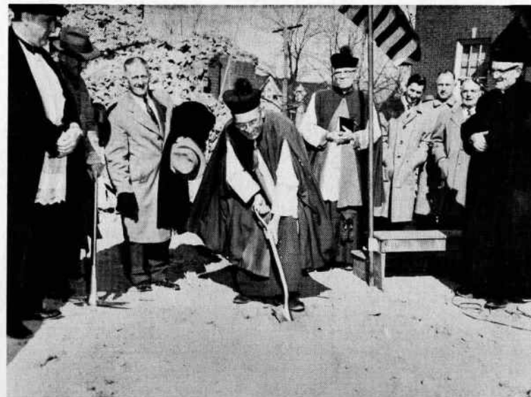
The First Shovel Of Earth
