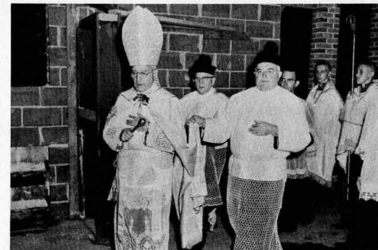
Bishop Klonowski blesses the foundation of the church. When the sprinkling is done, he says:
