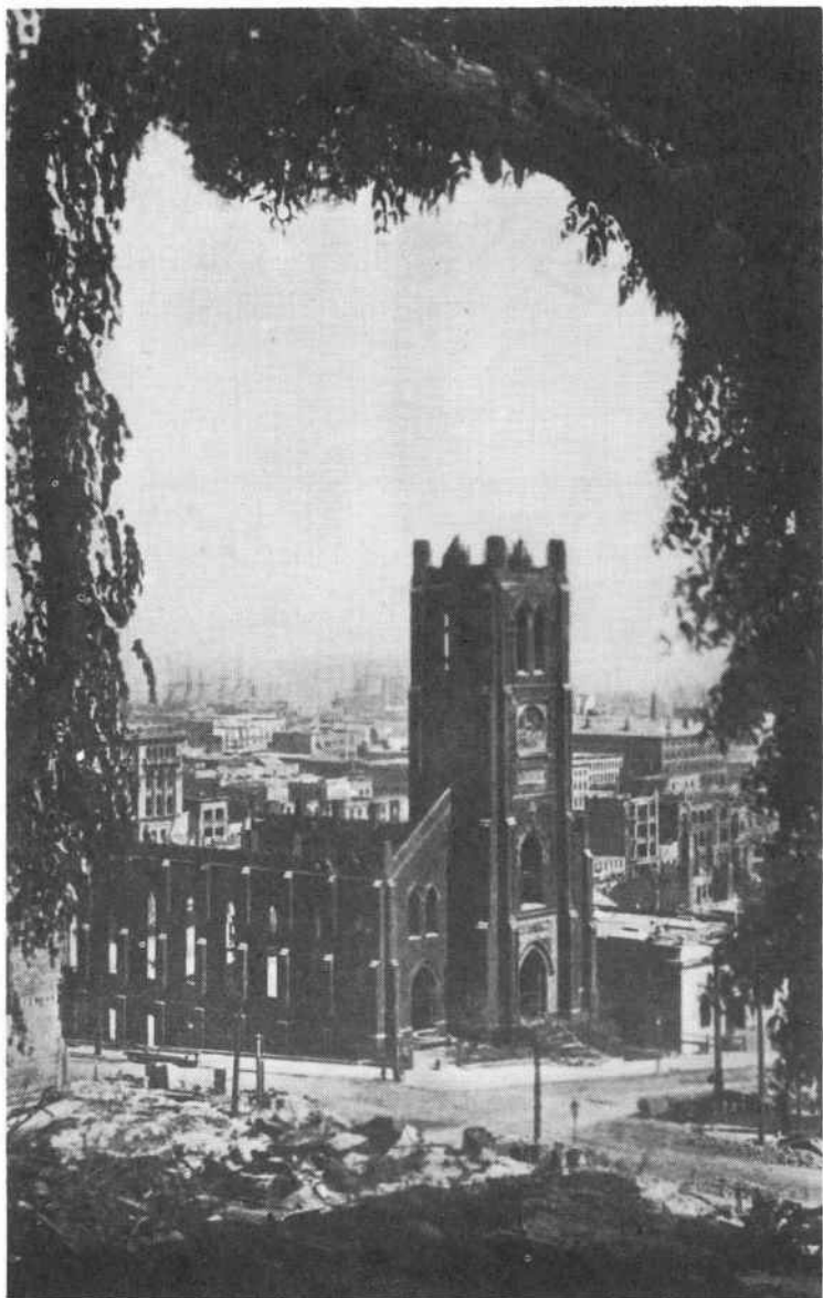
St. Mary's after the 1906 Earthquake Fire
