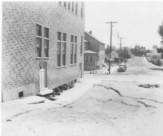
This old picture of the school shows the results of the cave-in caused by severe mine subsidence in the 1940s
