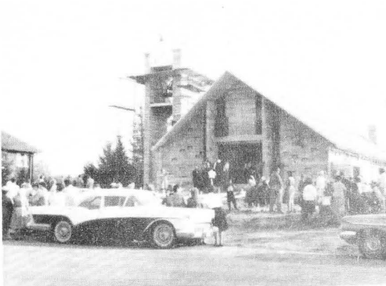
New Church Nearing Completion
