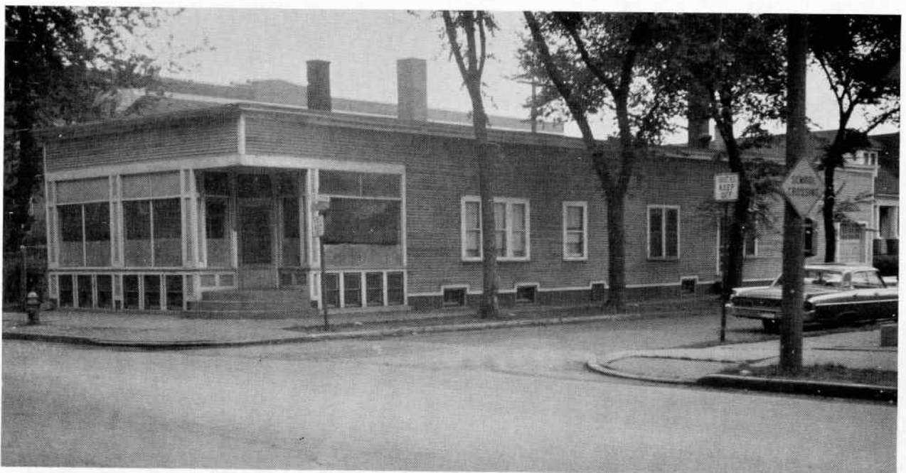
The first parish Mass was offered in this building on March 17, 1917
