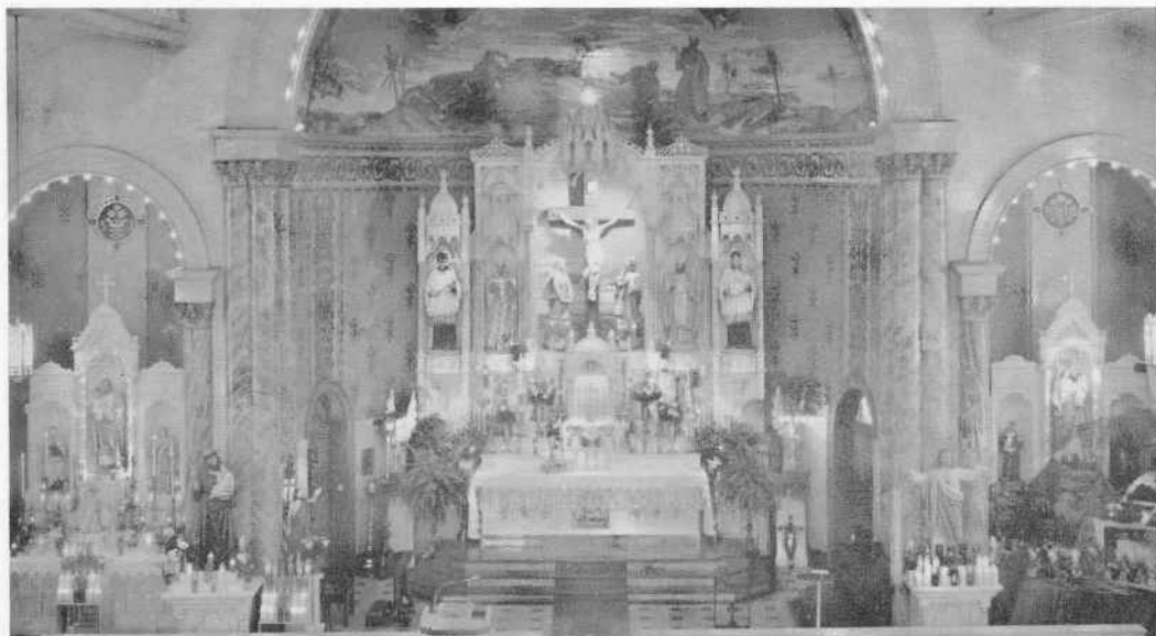
Church Interior around 1965
