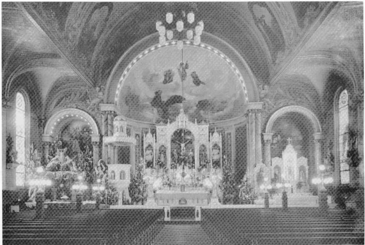
Church Interior around 1940
