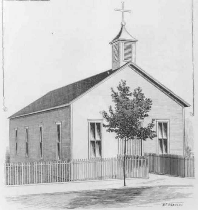
first polish church building in Mt. Pleasant then school
